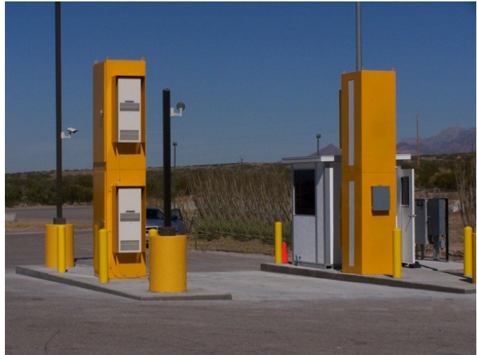
Figure 3 Installed HPGe Portal at Anthony, New Mexico
