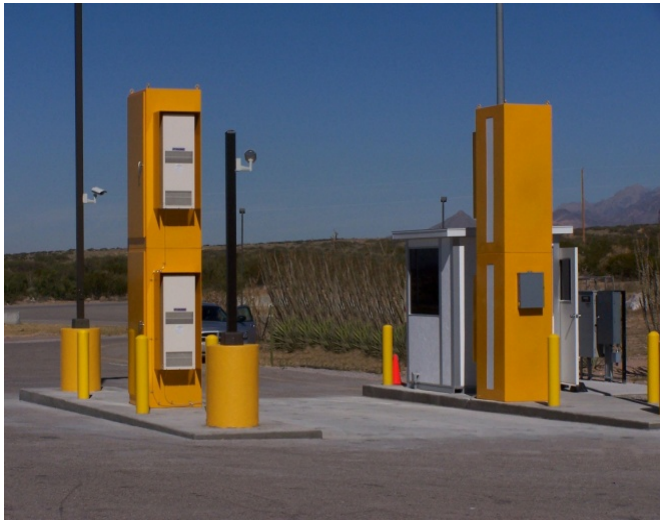
Figure 3. Installed HPGe Portal at Anthony, New Mexico. Figure 4. Typical installation of ARIS-1024 portal monitor.
